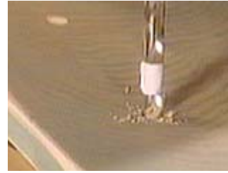
Drill the holes on the marks
