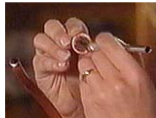
Apply flux to the washers and the pipe
