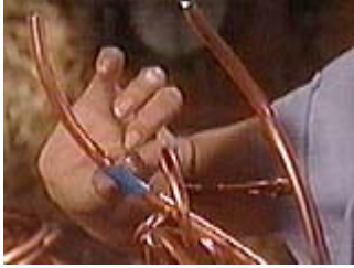
Mark the pipe that will carry the electrical wire so as not to drill into it
