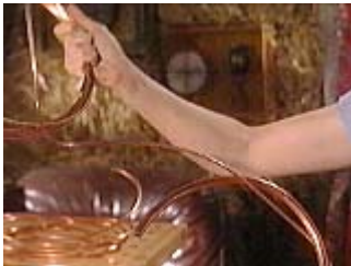
Twist the smaller tube around the main one and cut it off with a pipe cutter rasp to distress the corners and edges creating a worn look
