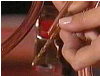
Select a drill bit the same size as the smaller pipe for a snug fit
