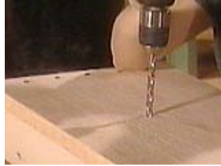
Drill a hole inside the letter
