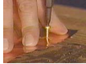
Use a hand screwdriver to drive the screws
