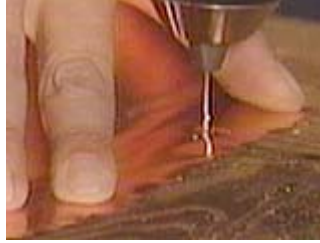
Drill prior to screwing
