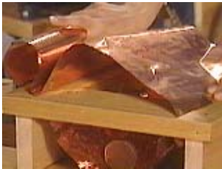
Place the copper foil over the opening to get a rough dimension for cutting
