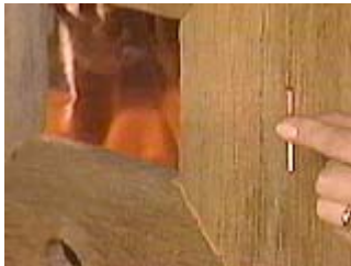
Use copper nails to attach the back supports
