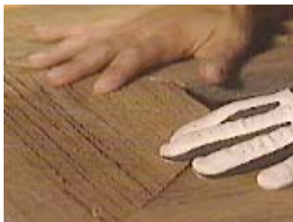
Fit the pieces together before gluing
