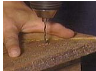
Pre drill before driving the nails in
