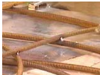
A proper weld contacts both pieces of metal that are to be bonded together
