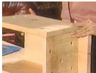
Drill four or five holes in the floor for drainage
