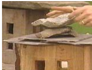
Cover the roof with a non-flammable material
