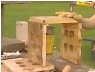
Nail the sides together
