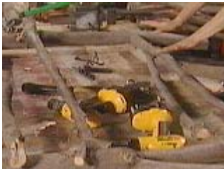
Lay out the pieces to be attached
