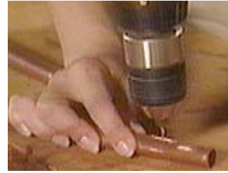
Drill a hole through both sides of the pipe
