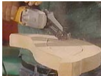
Cut along the base line with the mini grinder
