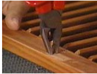
Use pliers to back out the headless screw
