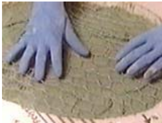
Place poultry wire on top of the mortar
