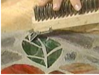
Scrape clean the surface of the glass and stone
