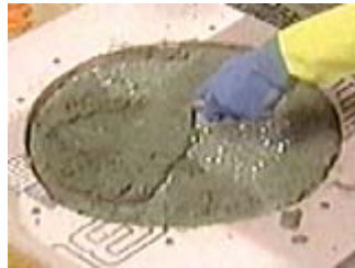
Fill the remaining space with concrete
