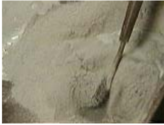
Mix up the mortar first
