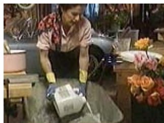
Use acrylic admixture to strengthen the mortar and the concrete
