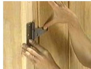
Attach hinges to the doors and the side trim
