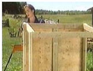
Use the plywood to square up the framing as you go
