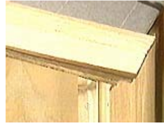
The two layers should overlap the front and sides by about half an inch
