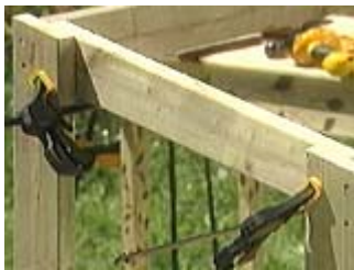
Attach using three inch zinc screws
