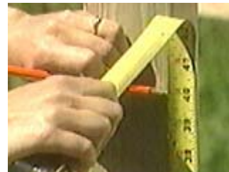
Measure the front post six and one half inches above the height of your garbage cans
