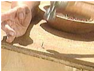
Attach the shingles with nails about 7 - 8 inches up from the bottom
