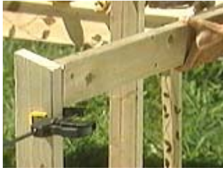
Use clamps to balance the boards while attaching them
