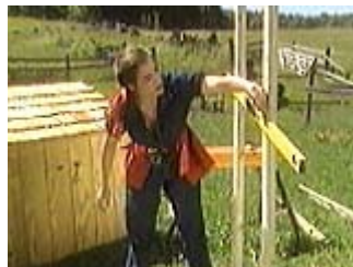
Mark the pitch angle on the posts and cut on the line
