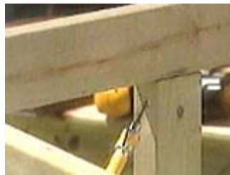
Toe-screw a center support to the back
