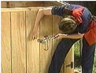
Attach closing hardware to the doors
