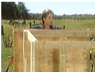
Cut and attach the plywood to the back and sides
