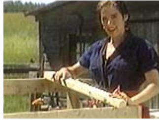
The angle for the rafters is the same as the one cut on the side posts
