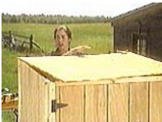
Cut a plywood top to overhang the sides and front by one half inch
