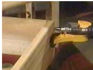
Pre drill for screws at the corners
