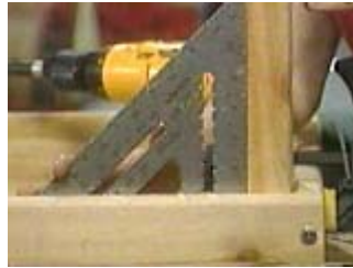
Use both a square and a clamp to hold the leg while installing the screws
