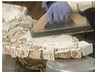
Work the grout in with the float
