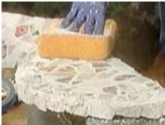
Always use a clean side of the sponge, and continually rinse the sponge in clean water!
