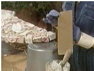
Use a rubber float to press grout into the spaces
