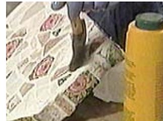
After curing, seal with grout sealant
