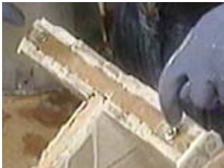
Drill and install screws for hanging the shelf
