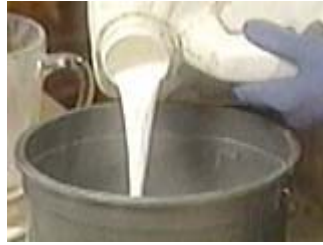
Use acrylic admixture for a stronger, more flexible bond
