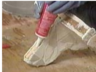
Seal the back with tub and tile caulk
