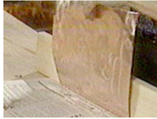
Lift the copper to start the bend
