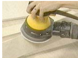
Sand the surface and the edges
