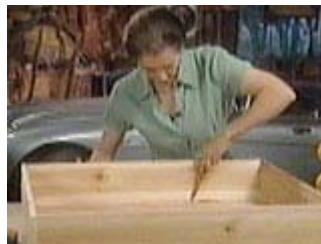
Mark the final flooring piece that will require cutting
