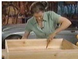
Mark the final flooring piece that will require cutting
