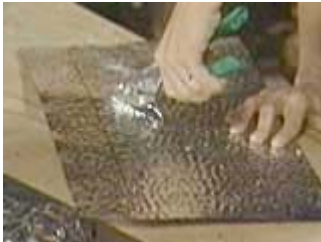
Then use tinsnips to cut out the centre section
