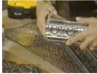
Cut the outside corners to fit snugly
