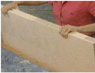
Attach a 2 x 4 or 2 x 2 along the top to support the 1 x 8 shelf
