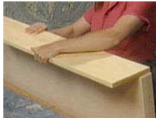
Attach a 1 x 8 shelf along the top
