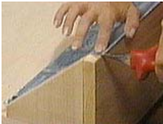
Round over any sharp edges with pliers...
