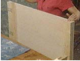
Attach 2 x 4s along the sides
