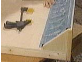
Cut out a triangular piece to cap the end of the crown molding
