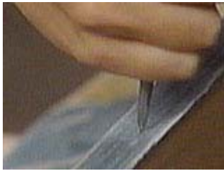
Use a nail set to drive the escutcheon pin flush
