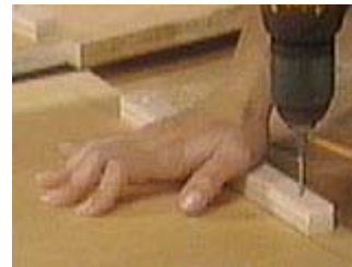
Finish off with screws for support
